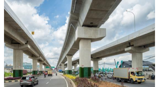
Road infrastructure project in Jakarta
