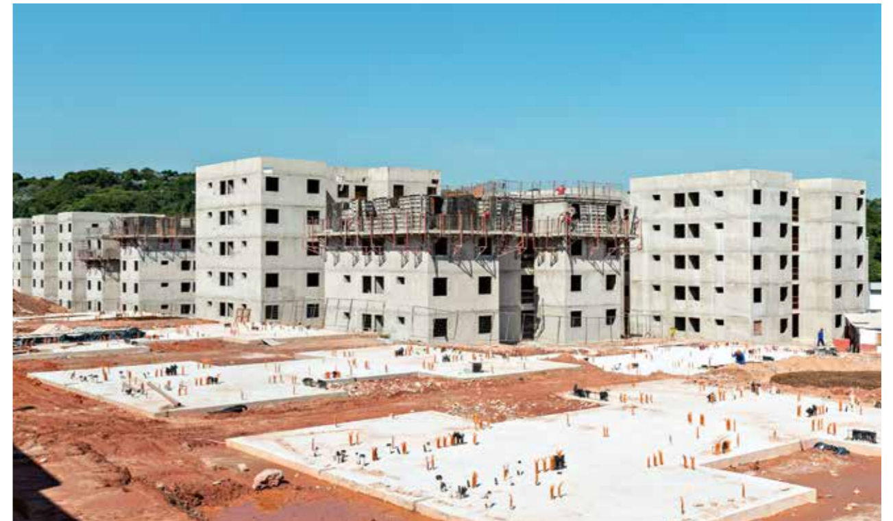
The average Direcional Engenharia construction project encompasses more than 1,000 residential units. The construction period for a residential block works out at 45 days, including interior finishing.
