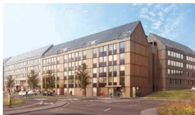
In the Swedish city of Piteå, Lindbäck is producing standardized components in Europe's most modern modular construction facility. Modular construction is frequently used in residential building.
