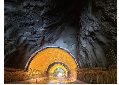
Kra Bao Tunnel, Thailand
