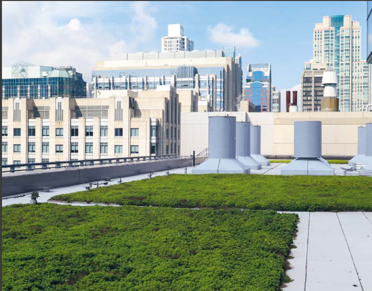
The acquisition of American Hydrotech makes Sika the market leader in the green roof segment in North America. The takeover fits perfectly with Sika's sustainability strategy. Photo: The green roof of Northwestern University's Simpson Querrey Biomedical Research Center in Chicago.
