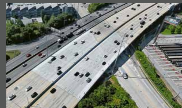
Following the collapse of the I85 road bridge in Atlanta, Georgia, Sika supplied its Sika® ViscoCrete® and Sika® Control-NS concrete admixtures to help complete the reconstruction a full month ahead of schedule.
