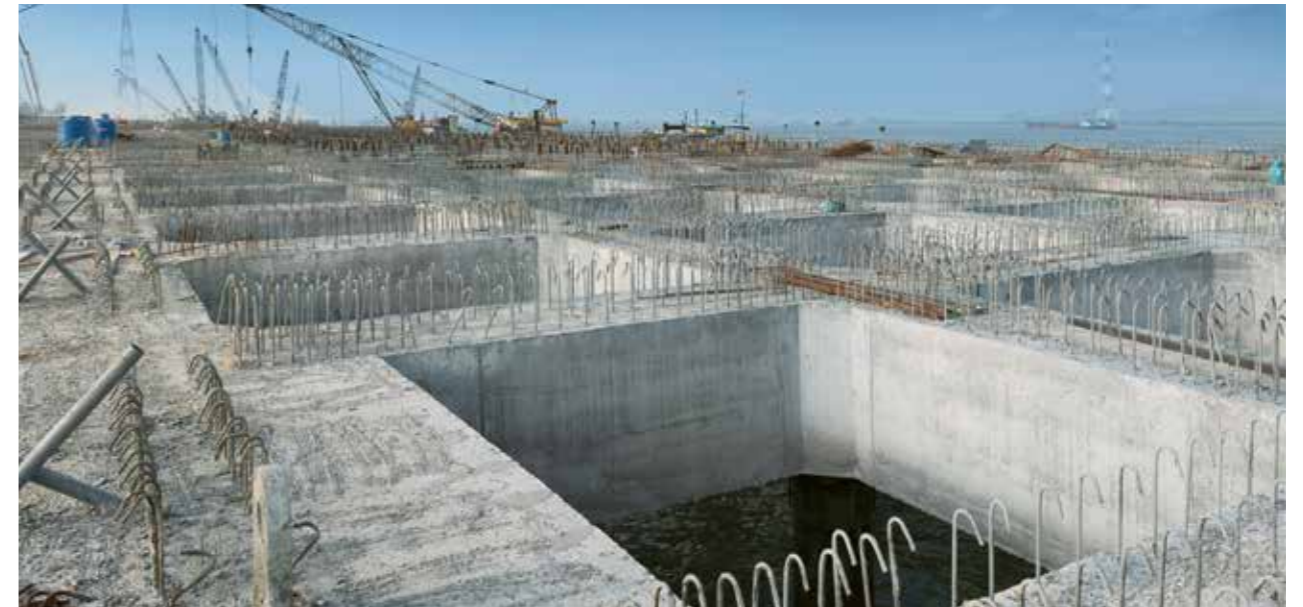
The Tan Vu Lach Huyen bridge opened in fall 2017 is the longest in Vietnam and part of a major port development project in the north of the country. Both the bridge and the forthcoming Hai Phong International Container Terminal include Sika concrete admixtures for high durability.
