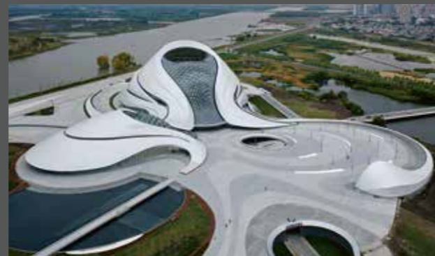
Recognized for its outstanding architecture, the Harbin Opera House in China was constructed using Sika products to help it withstand the harsh local climate.
