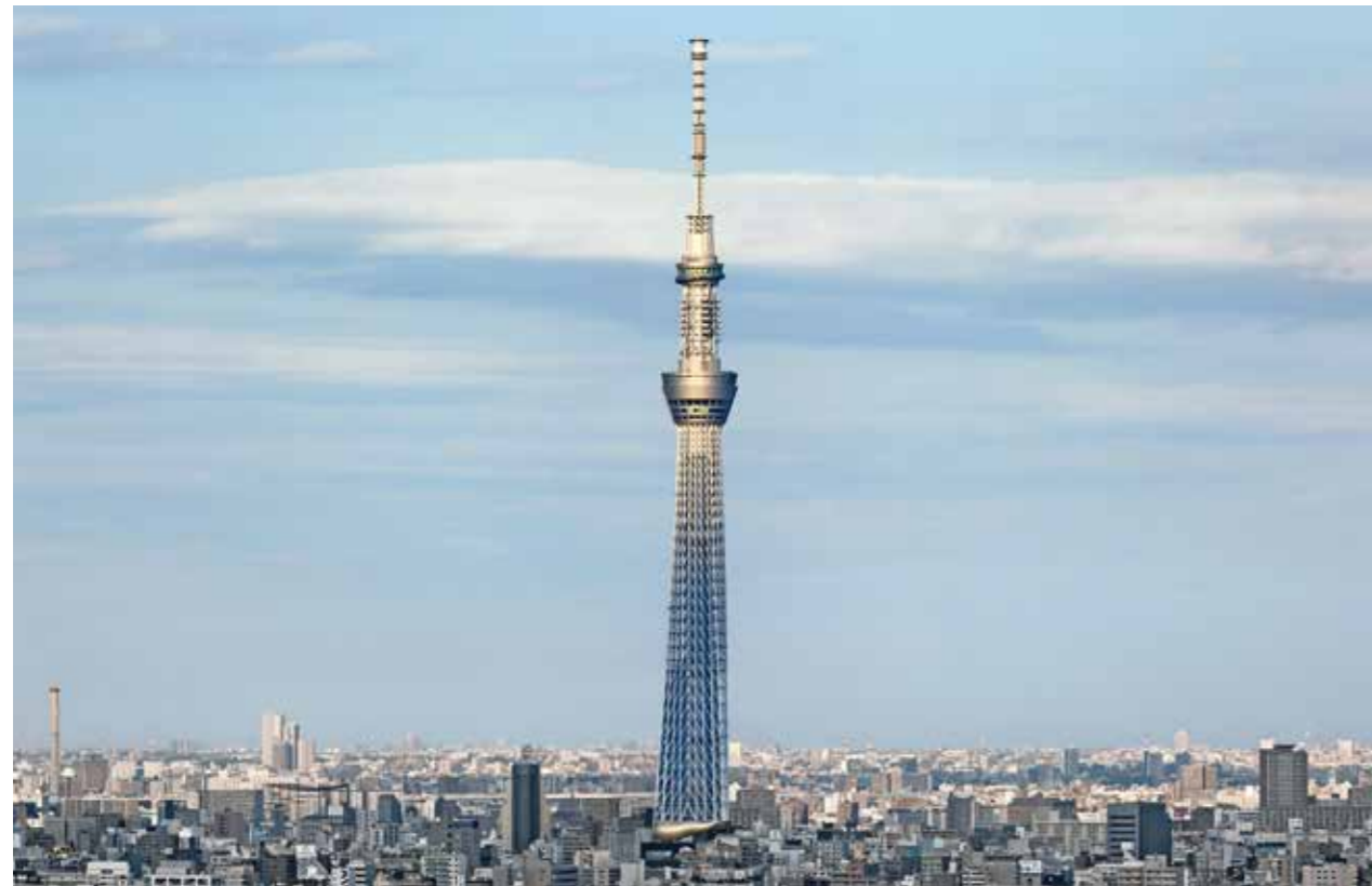
High-performance concrete superplasticizers from Sika were used in the 634-meter Tokyo Skytree, the world's tallest broadcasting tower. The construction time for Tokyo's showcase project with its central concrete pillar was just 6 months.
