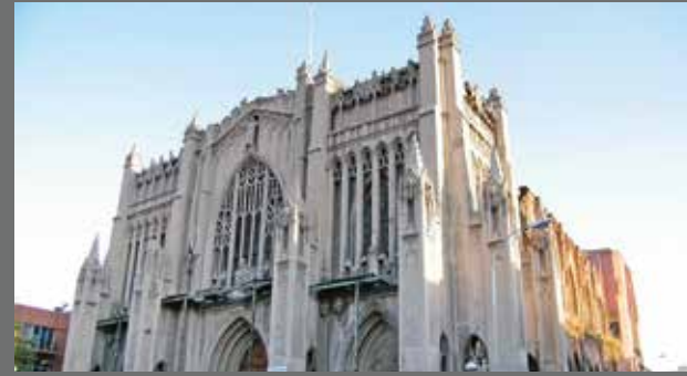
The historical basilica "La Basílica del Salvador" in Santiago de Chile built in 1874 was refurbished using Sikadur®-31, SikaWrap®-300, and Sikadur®-330. The basilica has a ceiling height of 30 meters and can hold up to 5,000 people.
