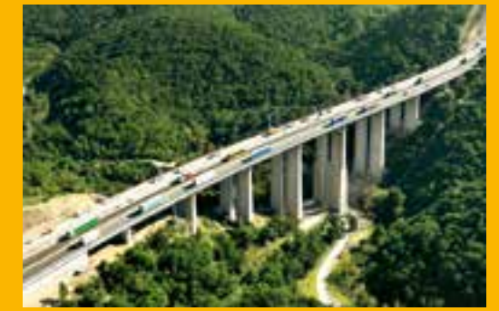
One of the challenges encountered while modernizing and upgrading the highway was strengthening the bridge piers in poorly accessible terrain.
