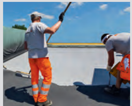
Priming, waterproofing, protecting and sealing. The Sika One Shot system makes coating parking decks a fast, simple and reliable process: installation rates of 1,000 m 2 per day are easily achieved.
