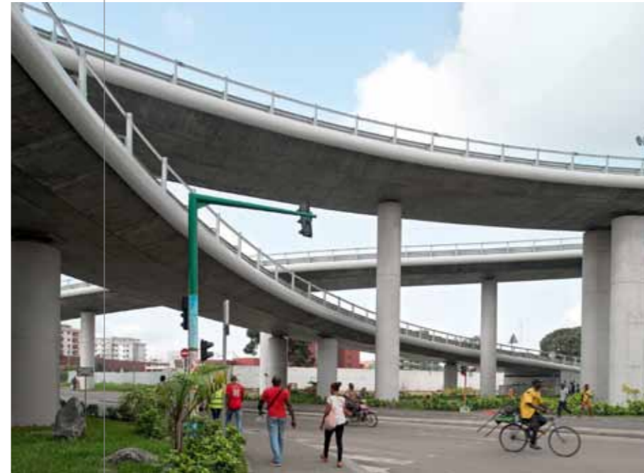
A bridge in Ivory Coast incorporating Sika products.
