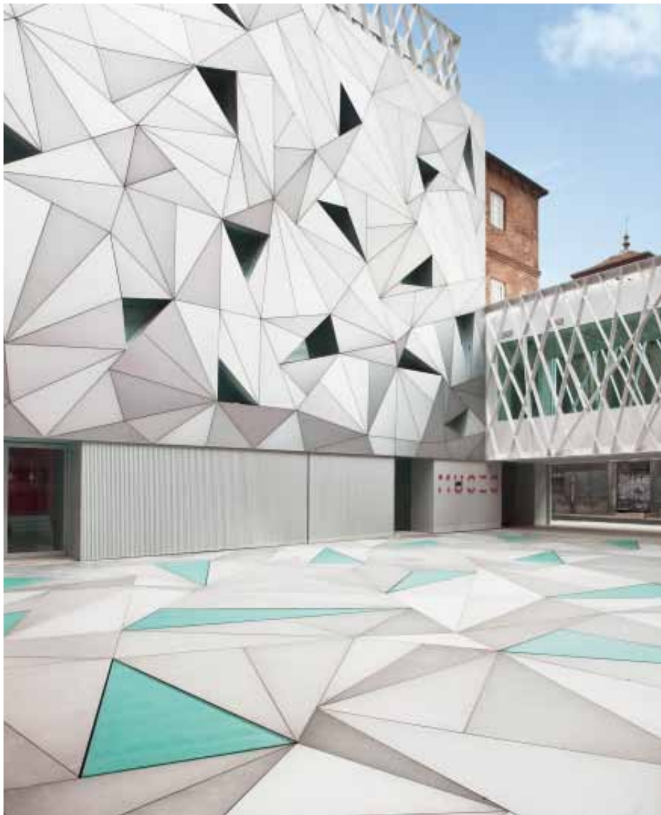
🕒 Elaborate composition at ABC Foundation museum in Madrid Although paving and façade are covered with the same aluminum tiles, two completely different Sika systems were used for their installation.
