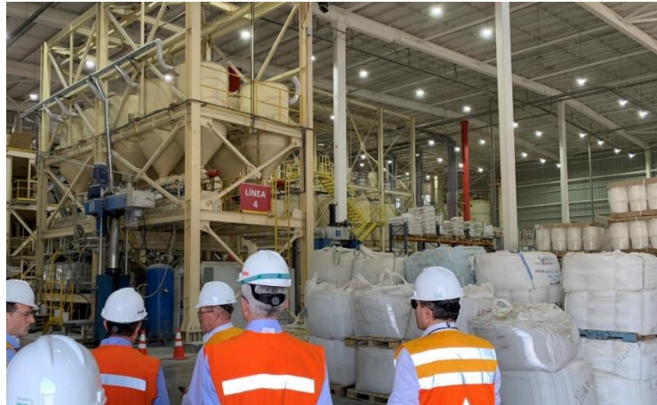
Parex Mortar Plant in Santiago, Chile
